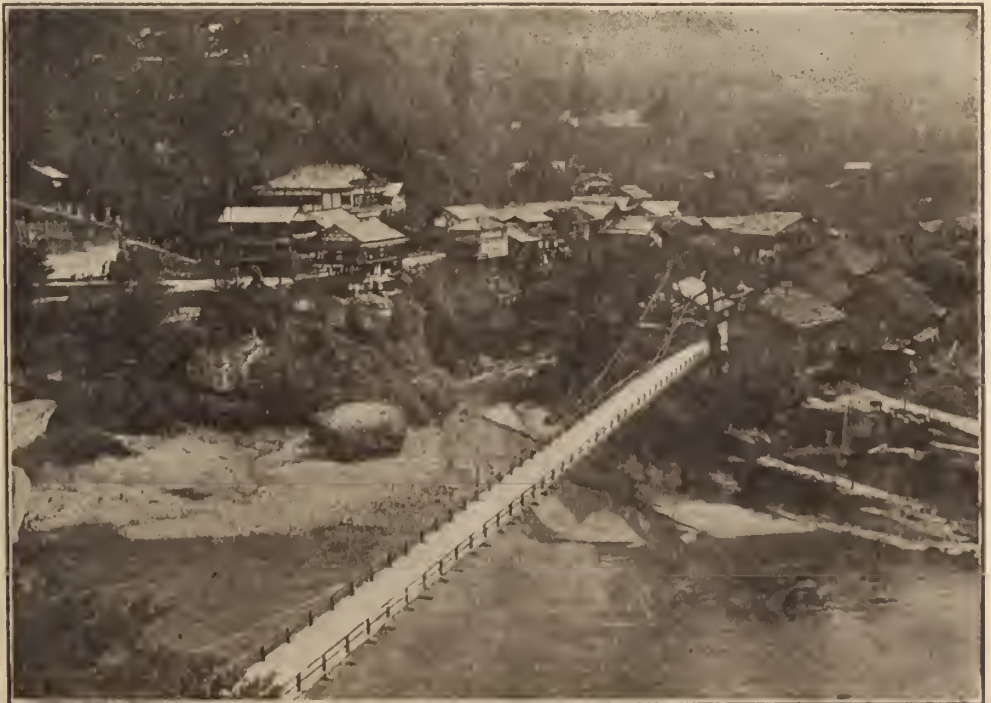
BRIDGE ACROSS TADAMI RIVER AT YANAIZU
